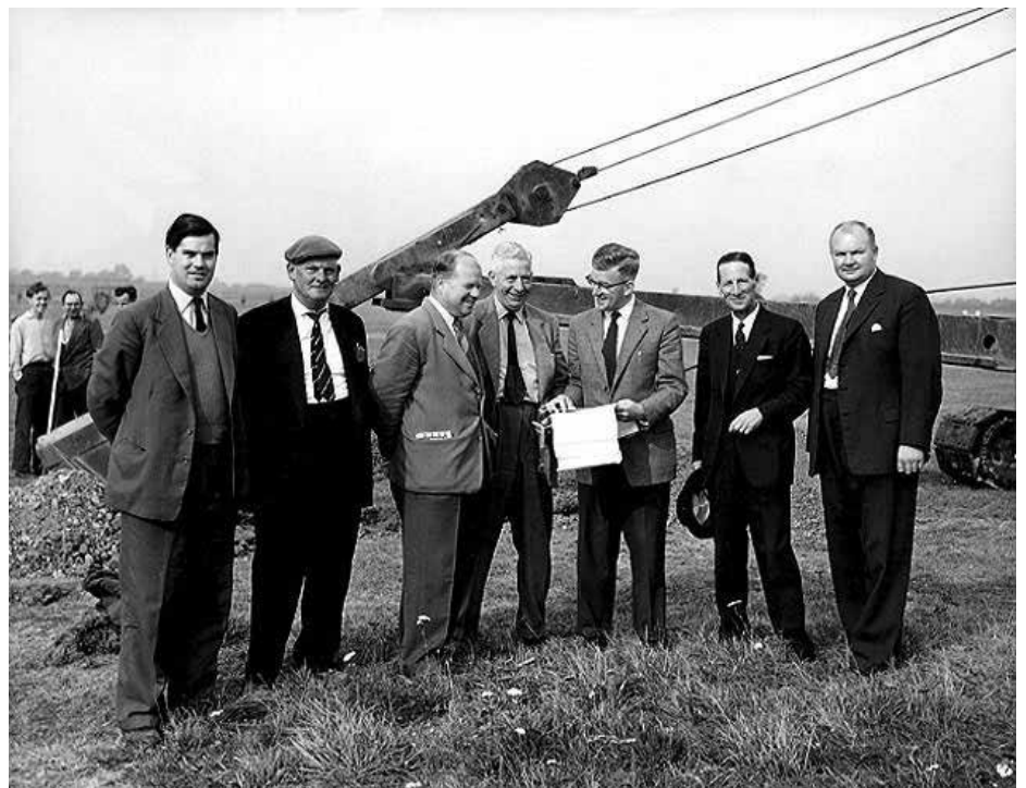
The team supervising the pipeline construction, Steve Stephenson, SMBP Engineering Manager, with the hat
